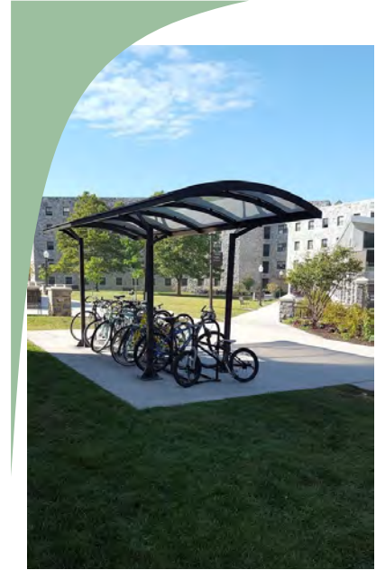
Covered bicycle parking.
