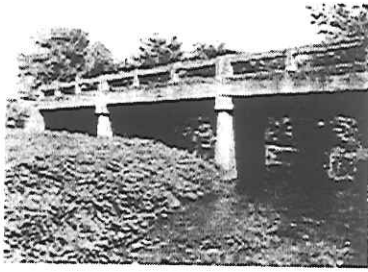
Stone Spring Road Underpass
