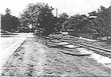
JMU Rail Road Corridor
