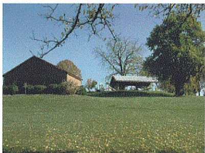
Restroom and Shelter (LPDA 2007)
