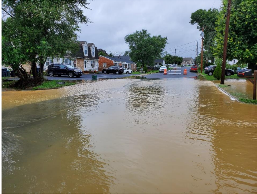
Figure 6: Photo 2 depicts September 1, 2021, flood extents on Suter St. on right side of the culvert outlet (facing downstream). Photo taken on 9/1/2021 at 1:28PM
