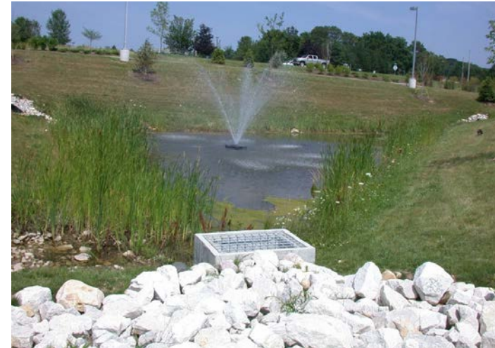
New developments require stormwater management such as ponds to hold and filter runoff.
