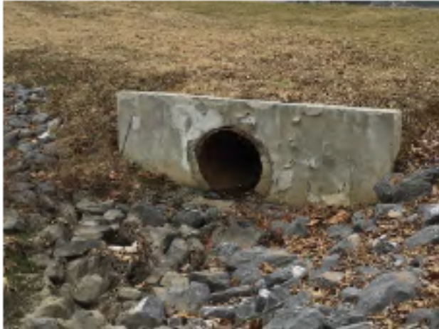
FIG 1: Trunkline E Outfall (36" SS)
