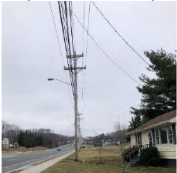
FIG 28: Reservoir Street at Foley Road (Facing South)
