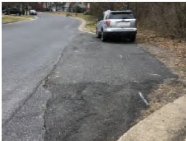
FIG 17: Curb Opening to Conveyance Channel at Woodland Drive (Facing West)
