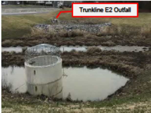
FIG 19: BMP 1 (Facing South)
