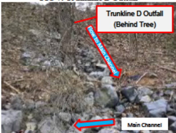
FIG 9: Trunkline D Outfall and Riprap
