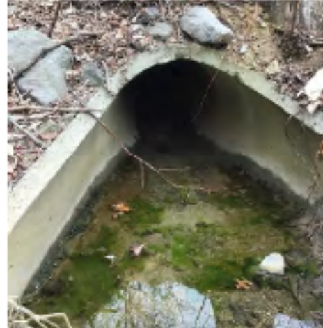
FIG 8: Trunkline B Outfall
