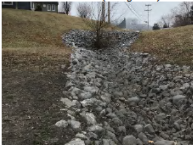
FIG 23: BMP 2 at Outlet Structure (Facing South)
