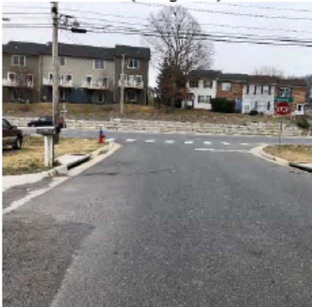
FIG 27: Intersection of Foley Road and Reservoir Street (Facing East)
