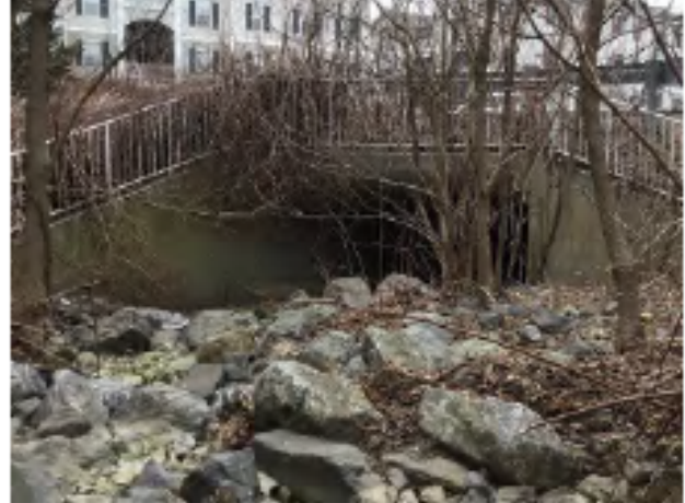
FIG 14: Ultimate Outfall of Project Limits (10'x6' Box Culvert Under Sunchase Parking)
