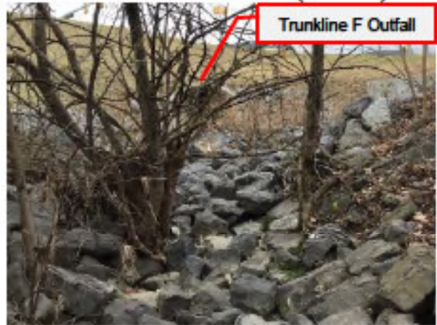
FIG 4: Existing Conveyance Channel (Facing Upstream)
