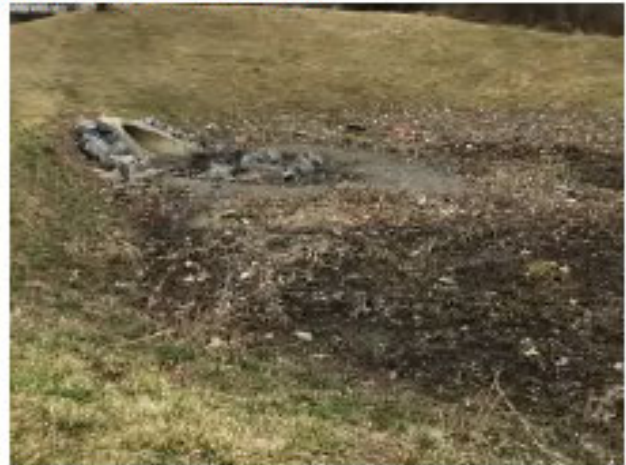
FIG 20: Trunkline E2 Outfall into BMP 1
