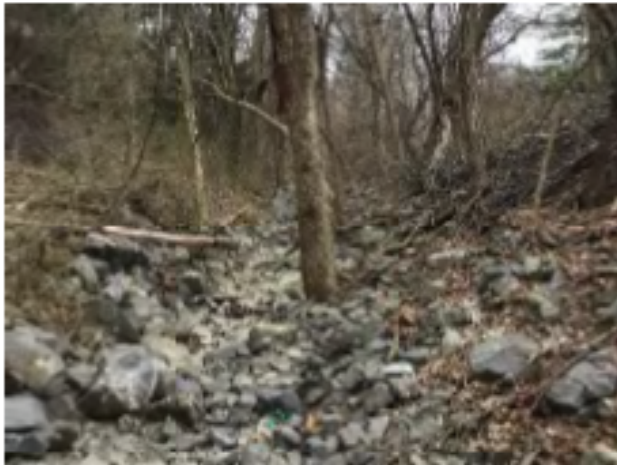
FIG 5: Existing Conveyance Channel (Facing Upstream)
