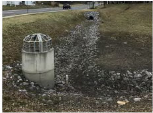
FIG 22: BMP 2 From Top of Berm (Facing East)
