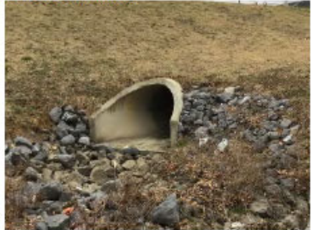
FIG 2: Trunkline F Outfall (60" RCP)
