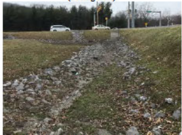
FIG 24: BMP 2 Basin and Outlet Structure, Facing Reservoir Street (Facing West)
