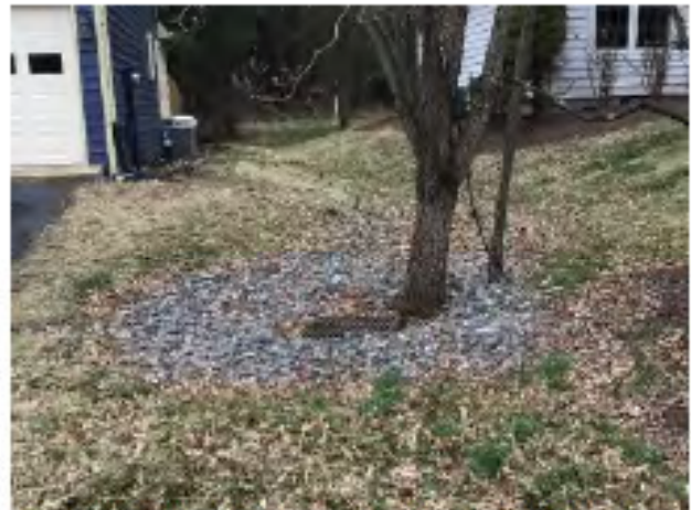
FIG 16: Yard Inlet and v-ditch at 652 White Oak Circle
