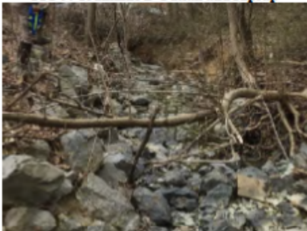
FIG 11: Existing Conveyance Channel, Upstream of Outfall (Facing Downstream)
