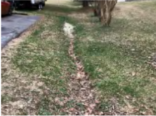
FIG 25: Drainage Ditch on 2210 Reservoir Street (Facing South)
