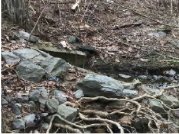
FIG 7: Trunkline B Outfall
