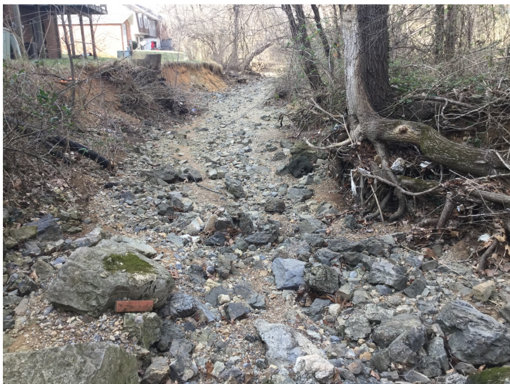
Figure 3-11 Looking downstream to eroded bank and large rocks within channel (10+00)
