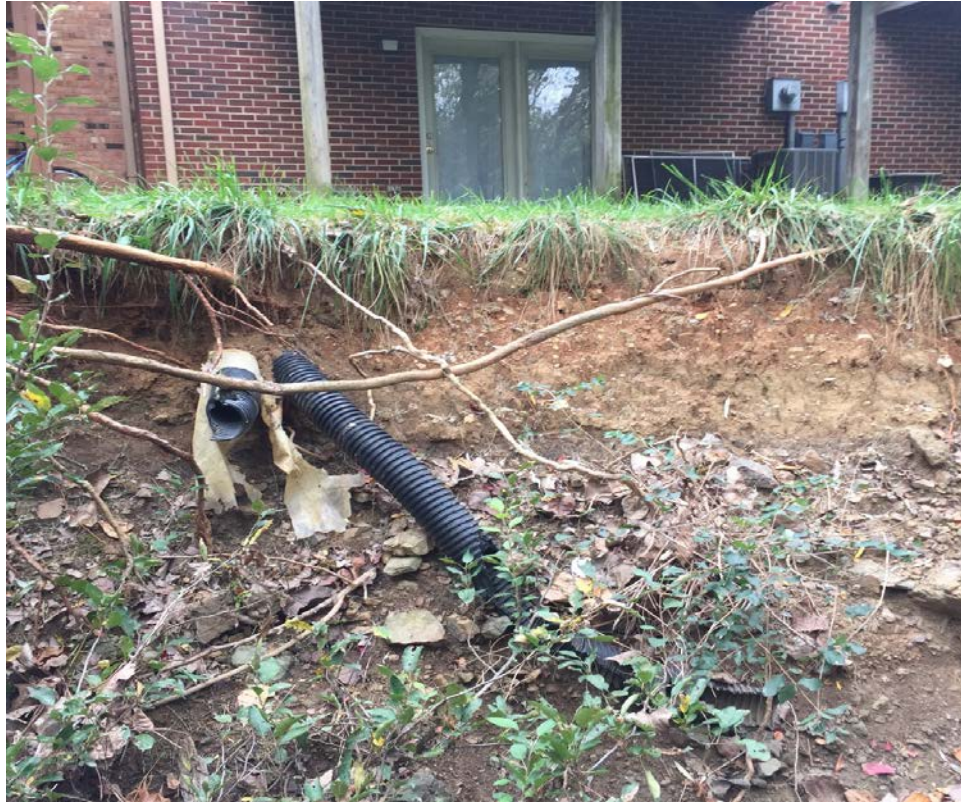
Figure 3-13 Exposed underdrain (9+50)
