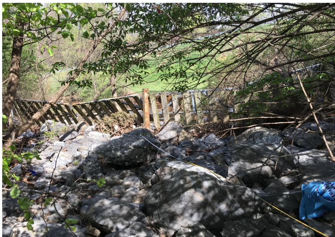
Figure 3-3 Looking Downstream Along Reach 1
