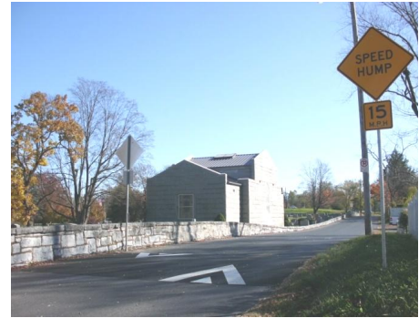
Example speed hump installed on a residential street.
