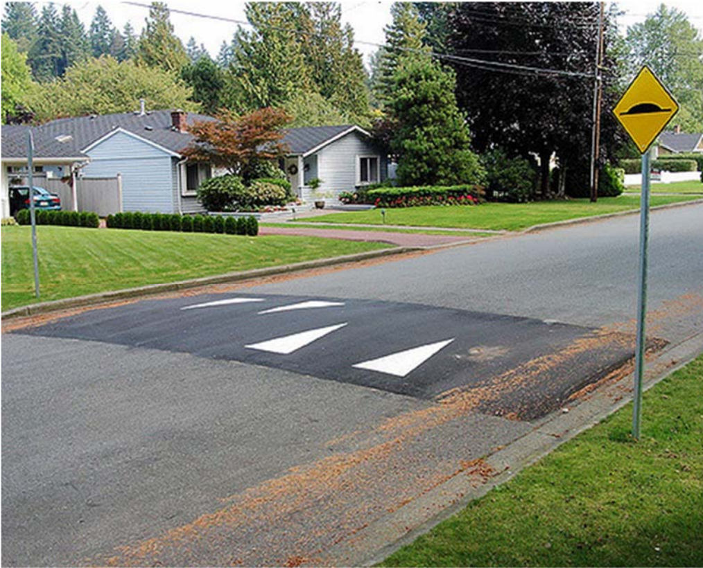
Speed Table – wide traversable speed hump, approximately 6" tall
