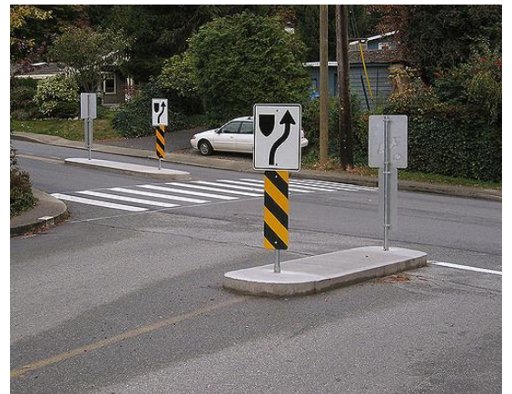
Traffic islands at stop sign
