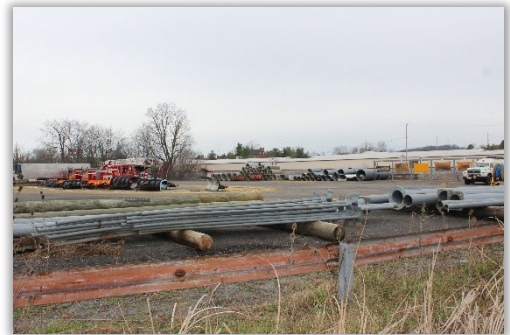
Photo 7: Outdoor material storage at the Public Works Facility.
