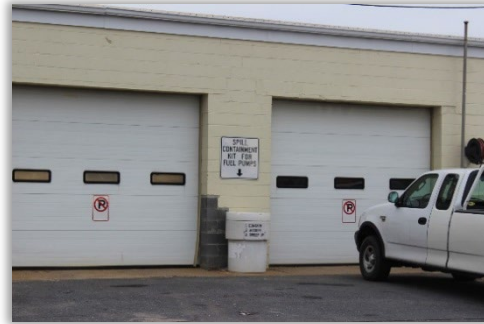
Photo 2: Spill kit at Public Works facility.
