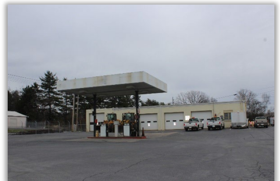
Photo 4: Fueling area at the Public Works facility.
