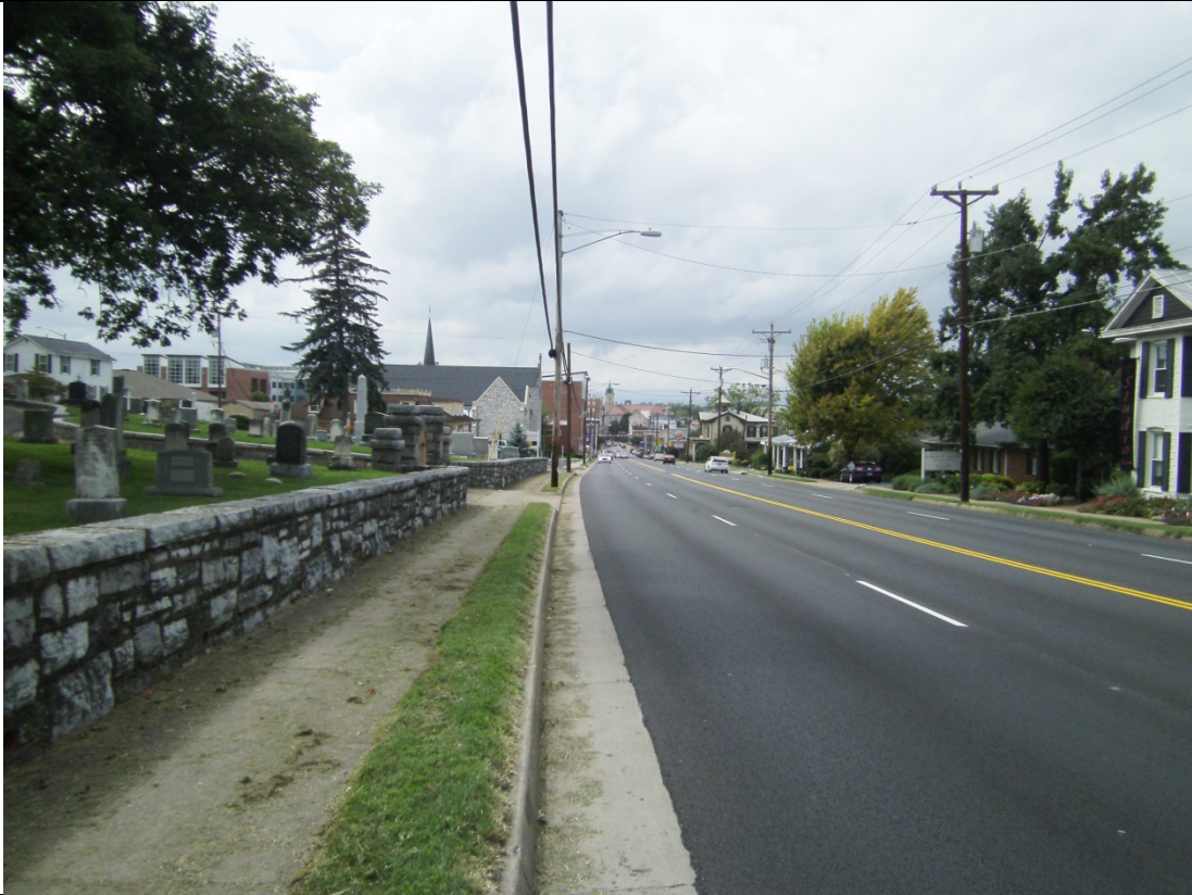
East Market Street before improvements (looking west from Myrtle Street)
