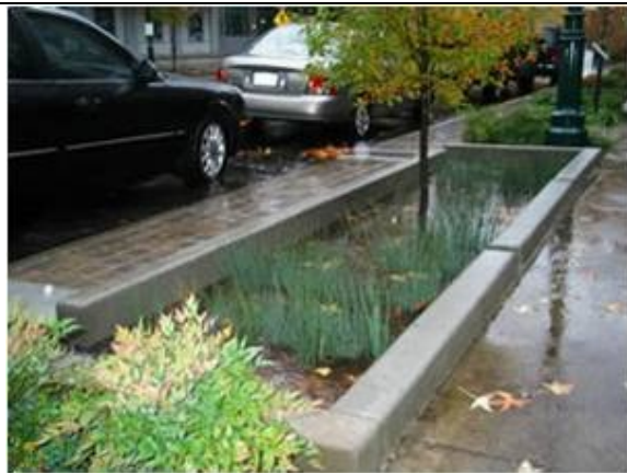
Planter boxes: Urban rain gardens with vertical walls and open or closed bottoms that collect and absorb runoff from sidewalks, parking lots, and streets.
