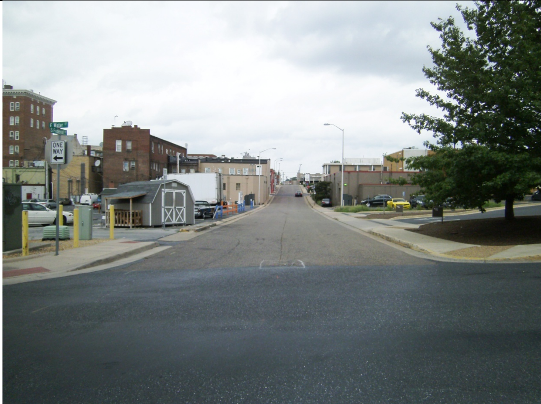
South Federal Street before improvements (looking north from East Water Street)
