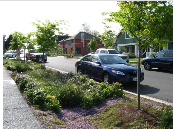
Bioswales: Vegetated, mulched, or xeriscaped channels that provide treatment and retention as they move stormwater from one place to another. As linear features, vegetated swales are particularly suitable along streets and parking lots.
