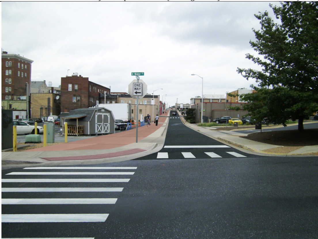
South Federal Street after improvements (looking north from East Water Street)
