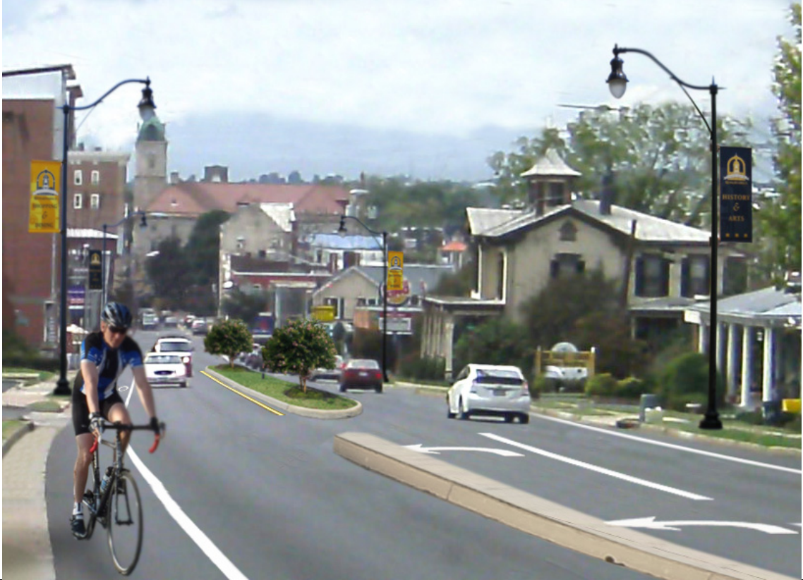
East Market Street after improvements (zoomed in, looking west from Myrtle Street)
