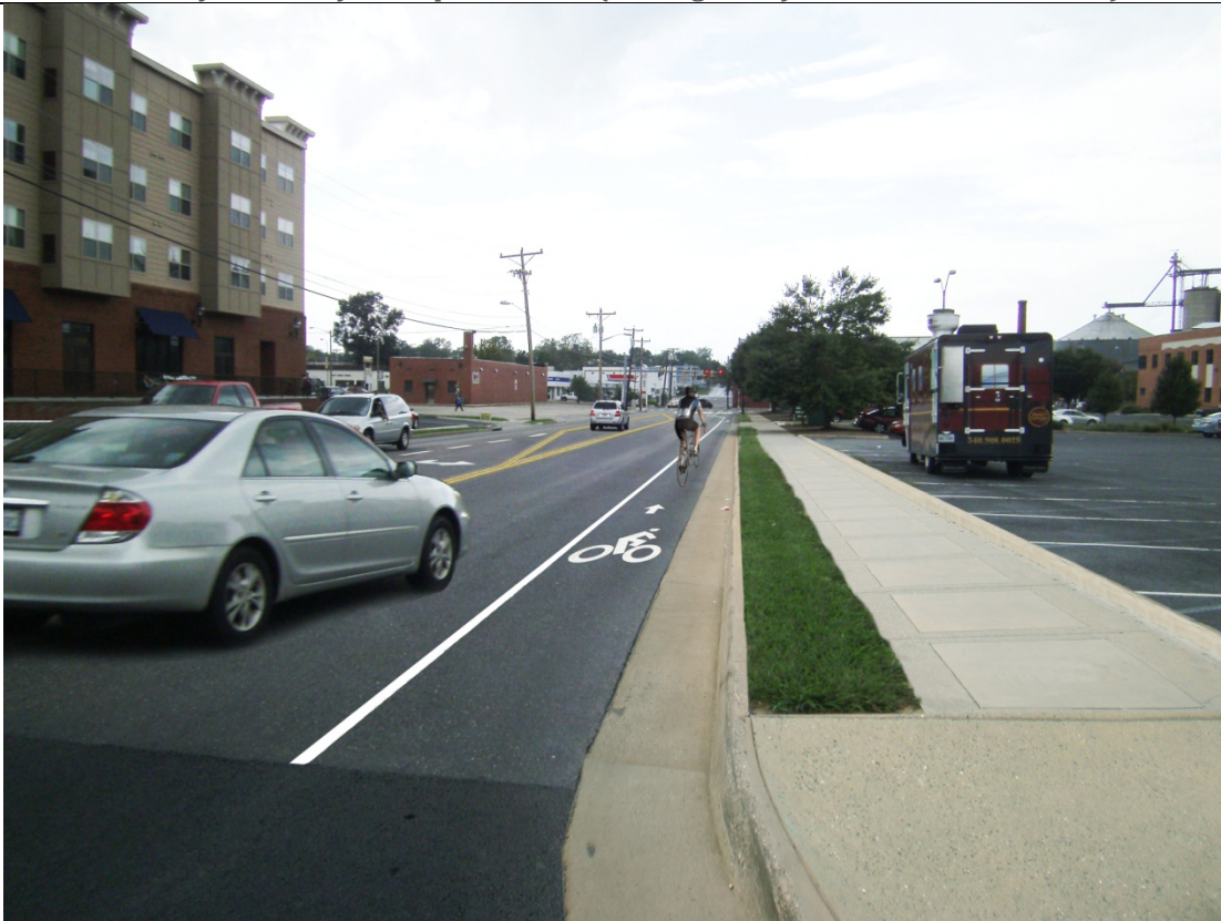
East Gay Street after improvements (looking west from North Mason Street)
