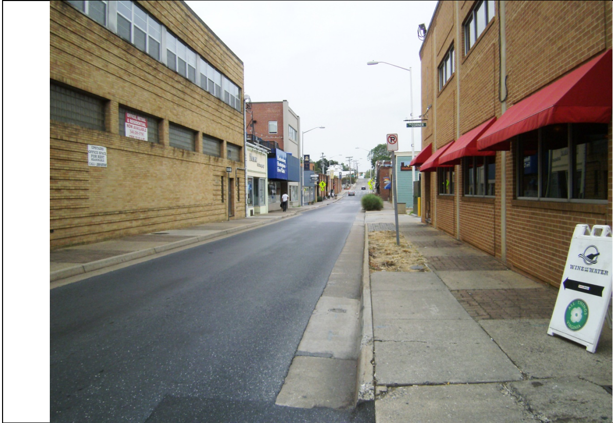
West Water Street before improvements (looking west from South Main Street)
