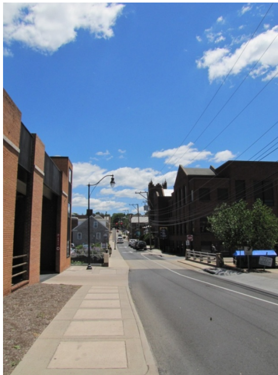
West Bruce Street after 2010 improvements
