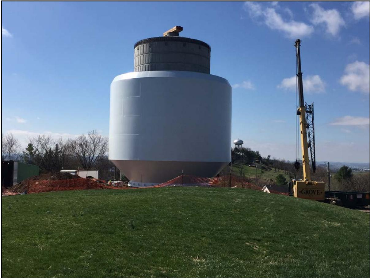
*Pictured above: A view of the water tank before it receives a final coat of paint and before the top of the tank is lifted into place.*
