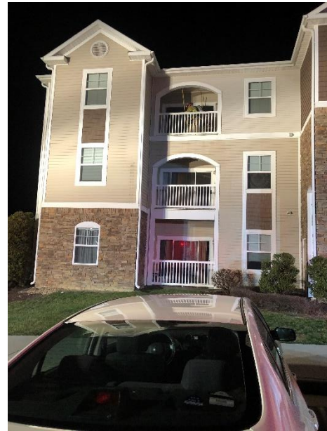
(Above) The fire started on a third-floor balcony and was controlled by a sprinkler.
