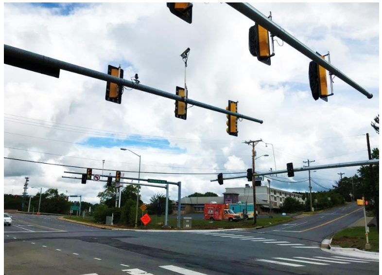
(Above) The new ramp is open at Port Republic Road and Interstate 81 North Exit 245.
