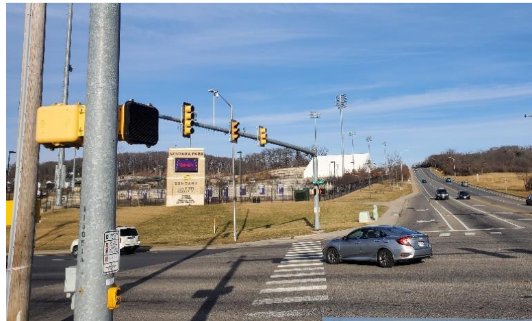
(Above) Signals at the intersection of Port Road and Neff Avenue/ Peach Grove Road. Work also will take place at the Devin Lane intersection.
