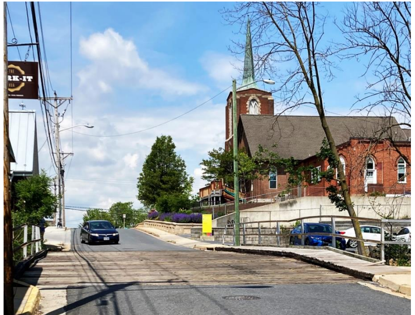
(Above)The Water Street bridge has closed for repairs.
