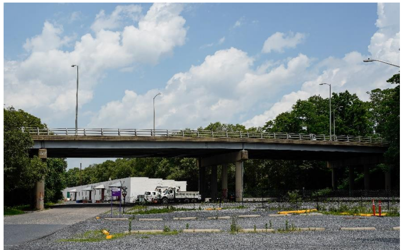
Crews will begin bridge work on Martin Luther King Jr. Way (above) between South Main Street and South High Street on Tuesday. Intermittent lane closures are expected for the duration of the project. Roads will remain open to traffic.
