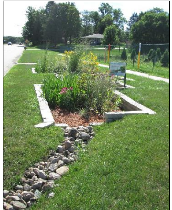
BMPs, such as bioretention facilities, help reduce excess nutrients and sediment in stormwater runoff.
