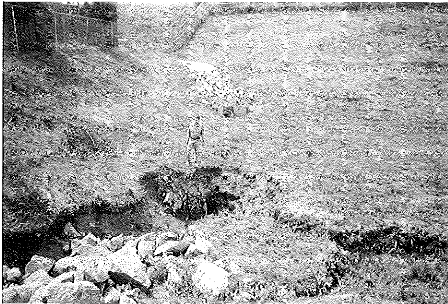
Figure 9.8. BMP Sinkhole Collapse
