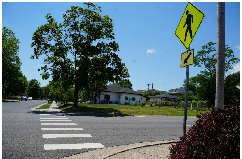
(Above) The crosswalk at Mount Clinton Pike and College Avenue. This intersection is part of the HSIP Crosswalks Project, which focuses on six different crosswalks around the community.
