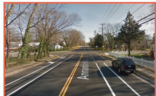
Annandale Road (After)
